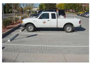
surge, and improve water quality. While completely functional, these paving stones appeared industrial, minimizing the aesthetic appeal typically associated with concrete pavers.
